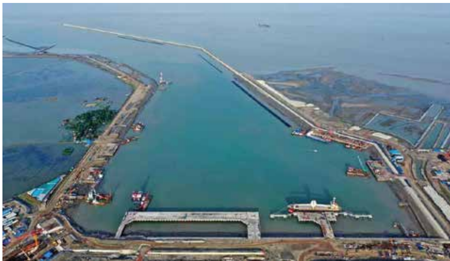
The concept of a deep-sea port in Matarbari emerged in conjunction with the government's coal-based power plant project in the area. The power plant required a wider channel and a port to receive fuel imports.
